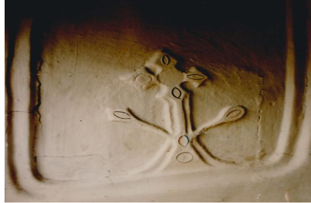
Figure 9 Wall of a house of a Kurmi family, Bardela, near Dhamdaha, Purnea
